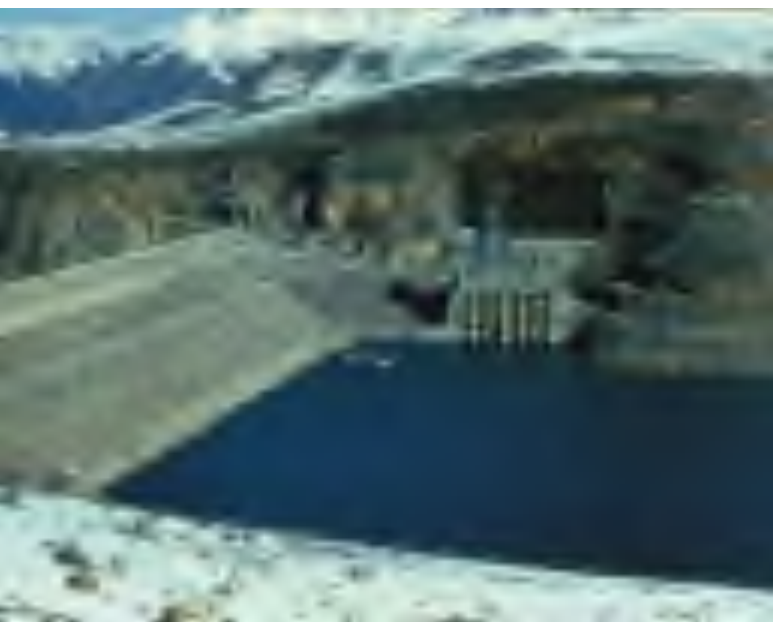
Charvak Hydroelectric Power Station (on the left – the upper reservoir with a storage capacity of 2,006 million cubic meters; on the right – the lower channel with a view of the dam, 168 meters high, and the powerhouse building)
